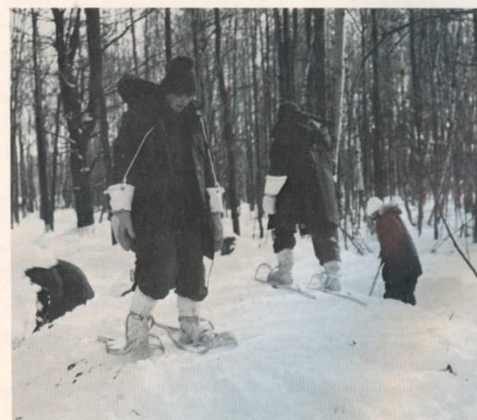
Pte Meade condenses surface snow during construction of a snow cave
